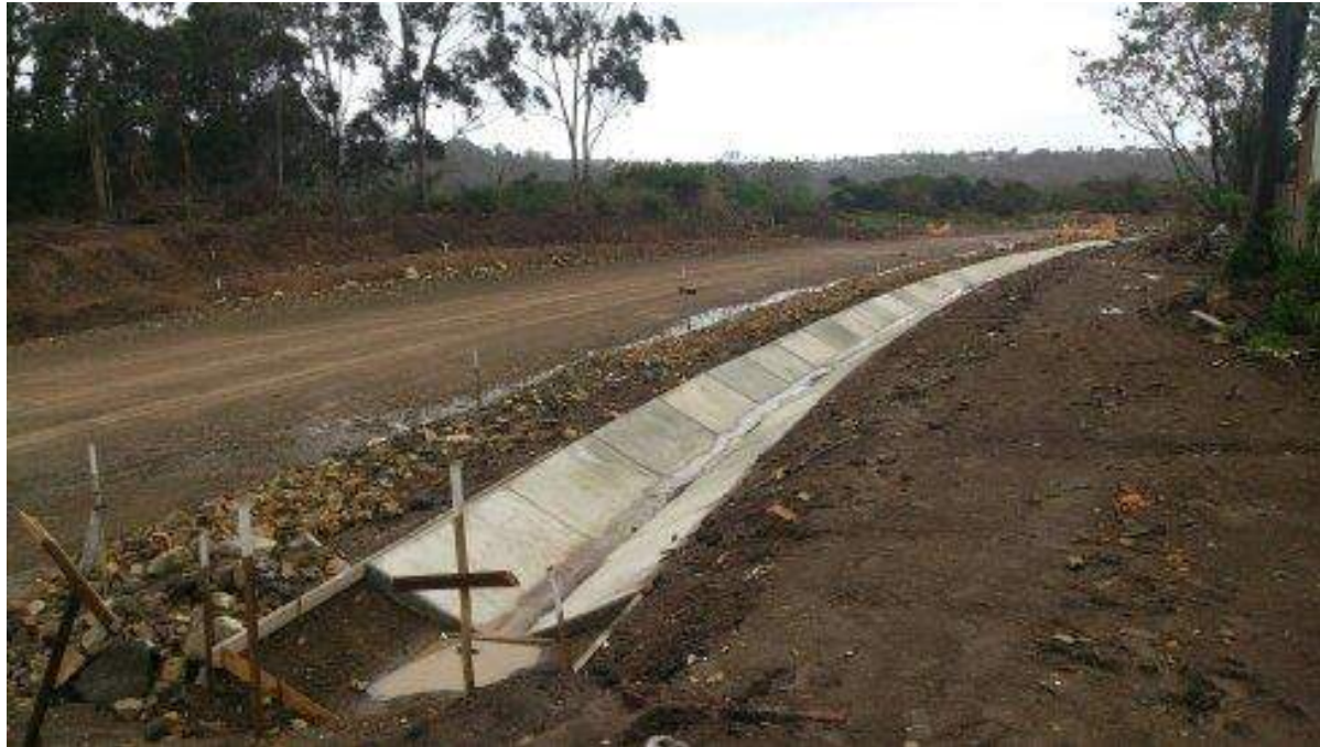
Above: Concrete V drain
