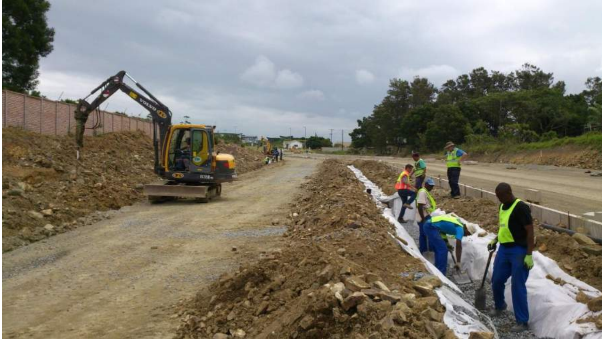
Above: Instillation of a subsoil drain
