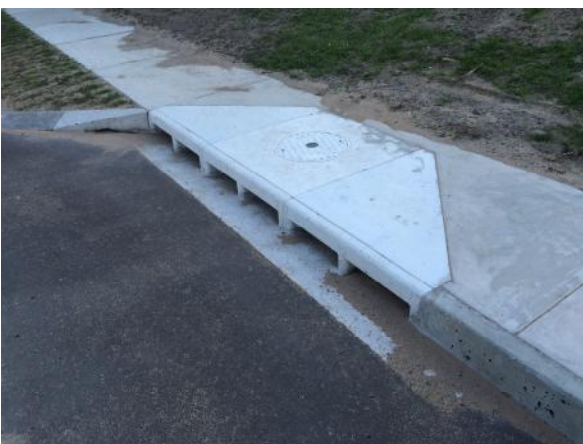
Above: New Polymer Kerb Inlet
