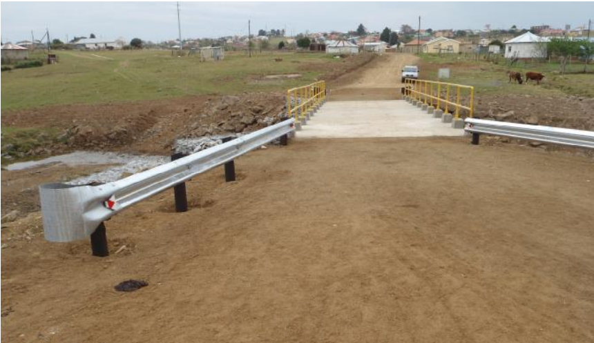
Figure – Ndevana Stream Crossing
